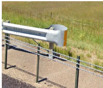
MGS Midwest Guardrail
