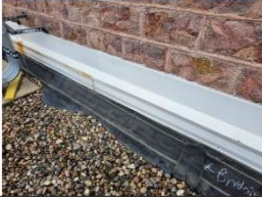
Bridging typical on this section
